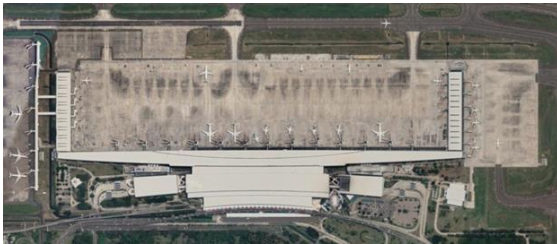
Gambar 6. Gambar Satelit Terminal 3 Bandara Soekarno-Hatta
