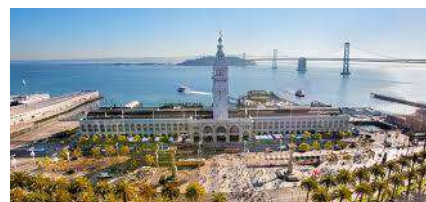
Gambar 3 San Francisco Ferry Building
