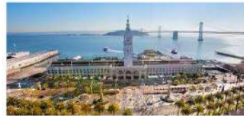
Gambar 3 San Francisco Ferry Building
