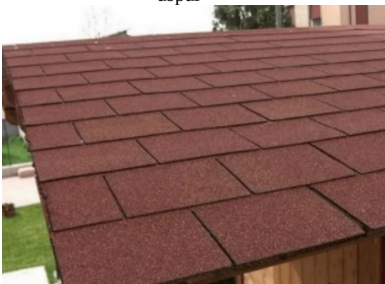
Gambar 106. Atap bitumen aspal
