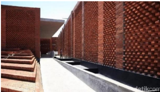
Gambar 104. Dinding batu bata expose
