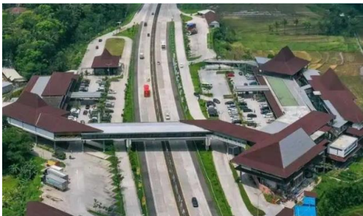
Gambar 105. Atap joglo bahan bitumen aspal
